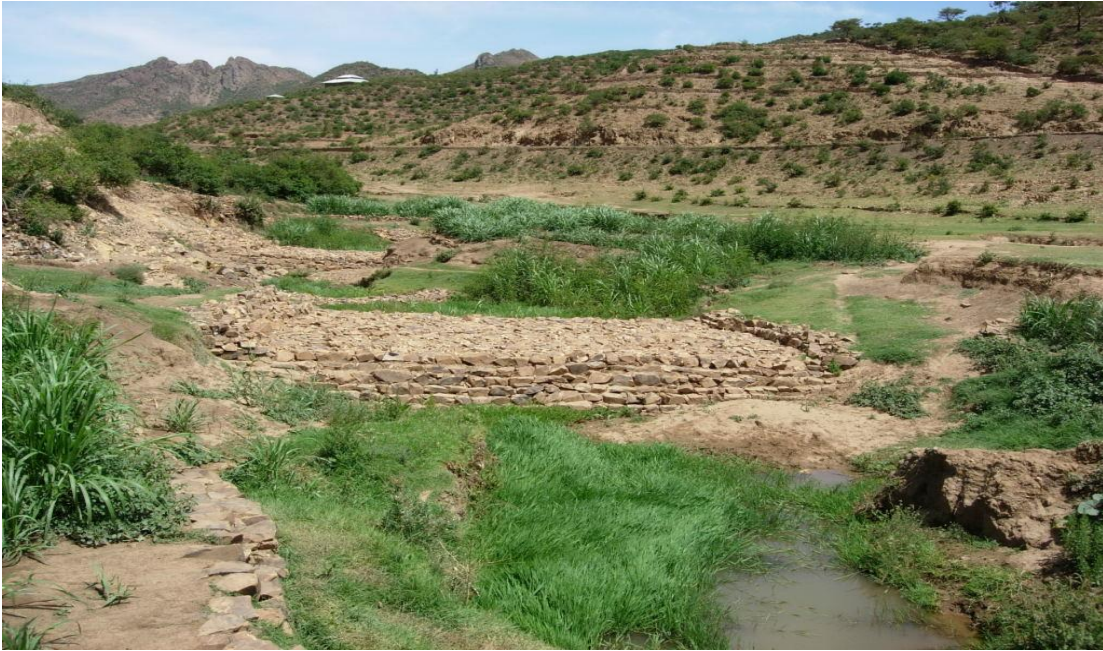
Fig 10 Stabilization of water ways and gullies
